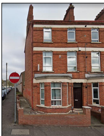
Figure 17. 43 Agincourt Ave, Belfast, UK
